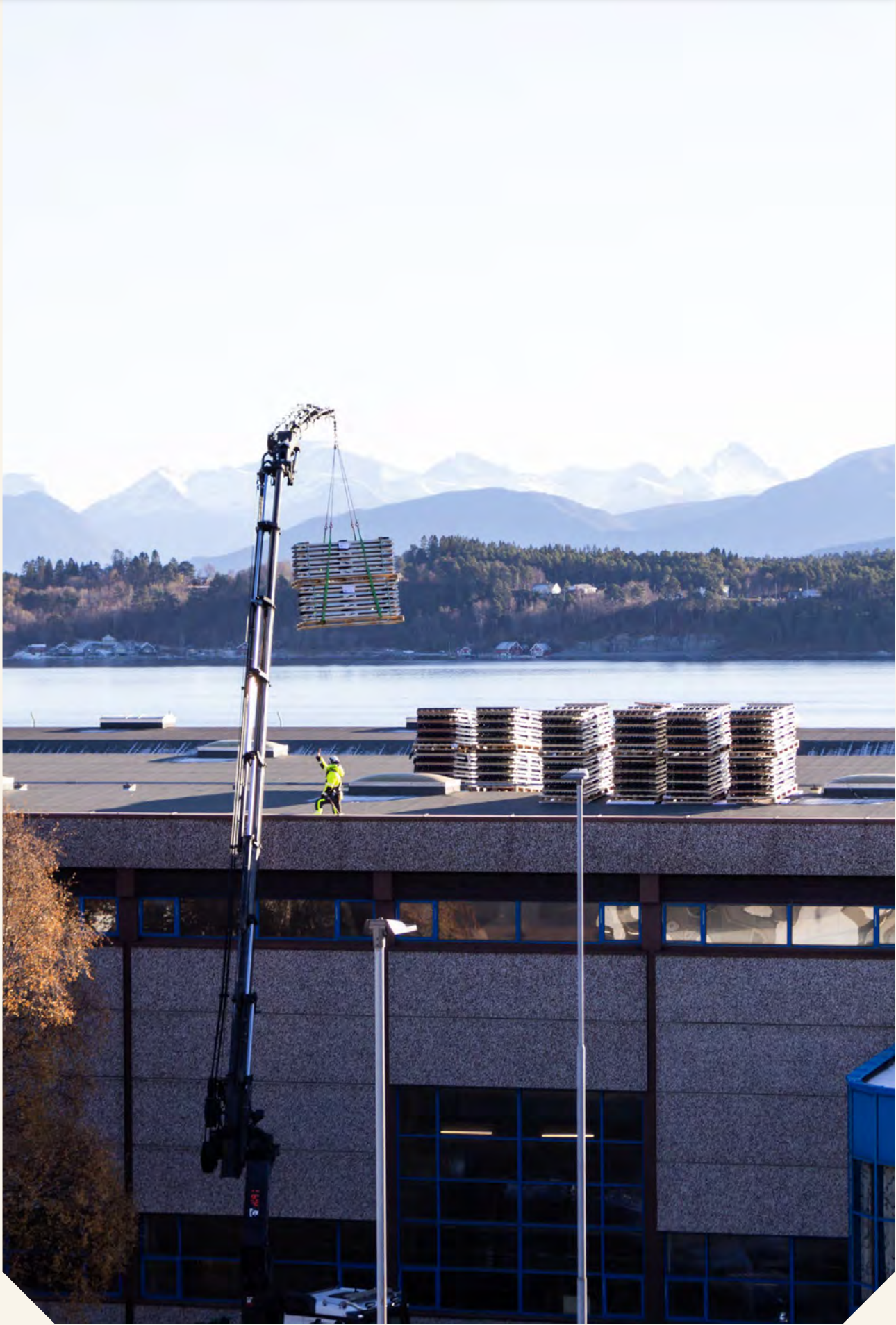
Solar panels being installed on the factory roof at Brunvoll in Molde.
